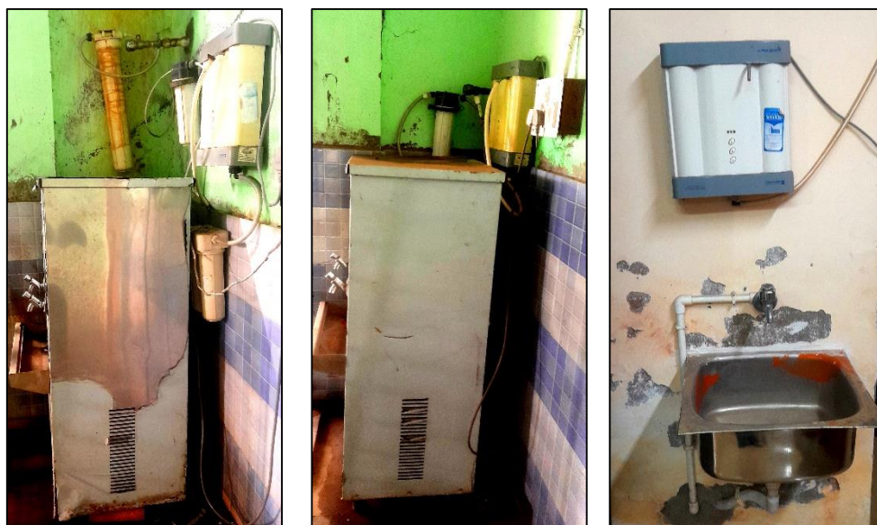
Figure 4: The filtered potable water units installed at Government General Degree College, Keshiary
